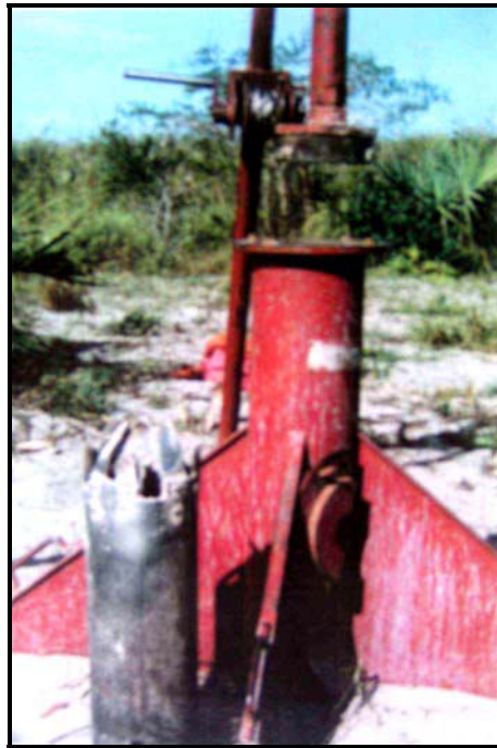
Figure 2.2 Photo Showing Vonder Rig Auger, Worktable, and Tripod Winch
