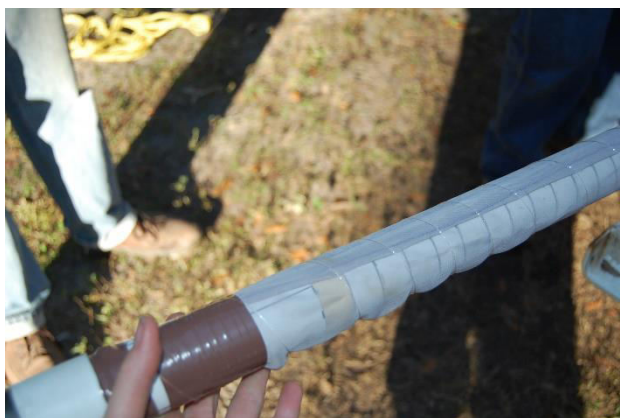
Figure 23. Completed Preparation of Wellscreen
