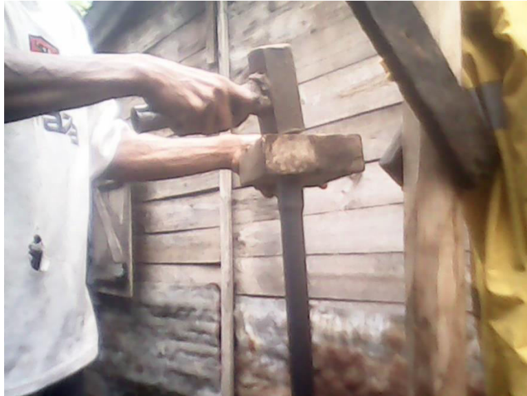
Figure 32. Hammering on PVC Pipe
