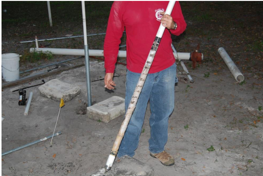
Figure 42. PVC Pipe after Drilling Well #9
