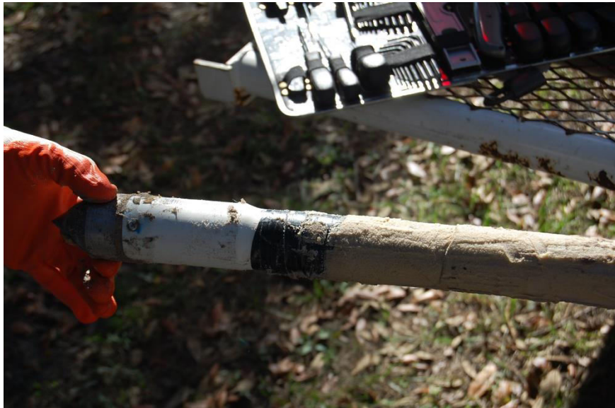
Figure 41. Exposed-Screen System B after Drilling Well #8
