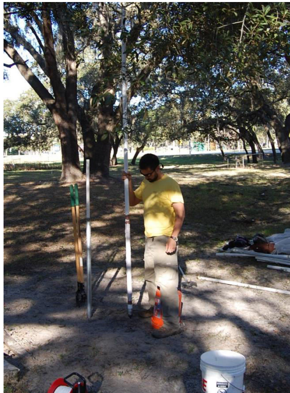
Figure 26. Finished Exposed-Screen System A
