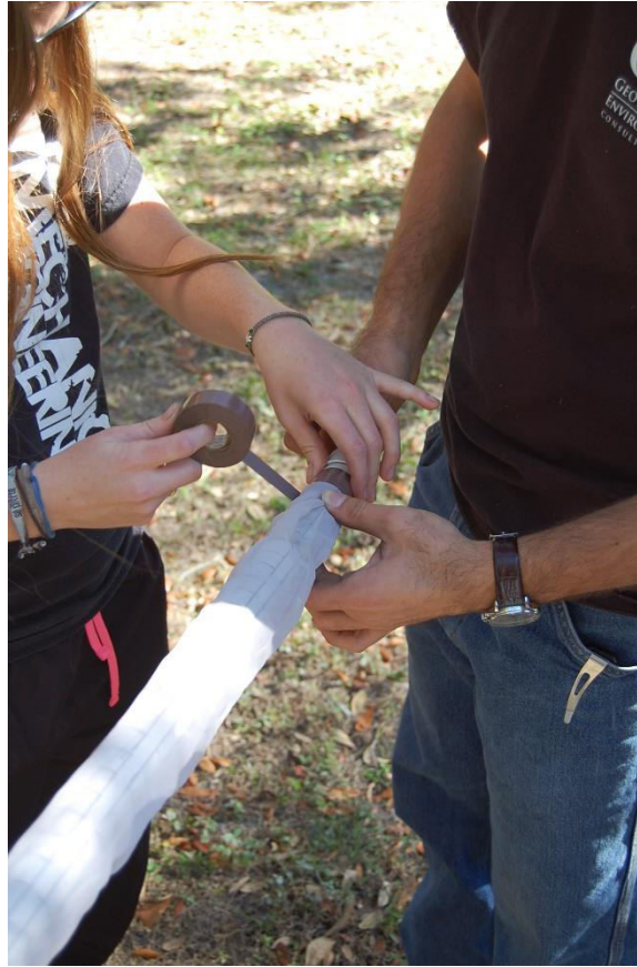
Figure 22. Preparation of the Riser Pipe
