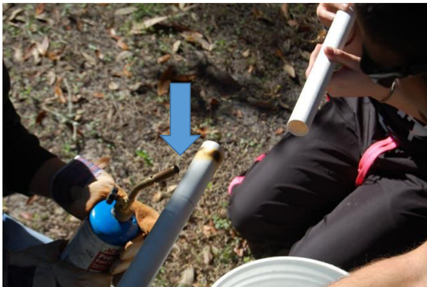
Figure 9. Heating a PVC Pipe
