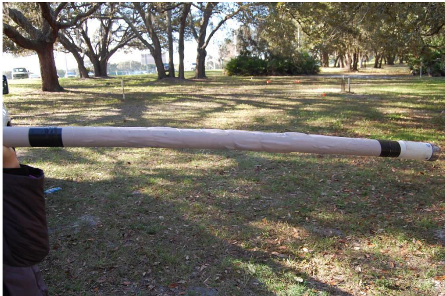
Figure 29. Schedule 20 PVC Pipe for Well #8 Prepared and Ready
